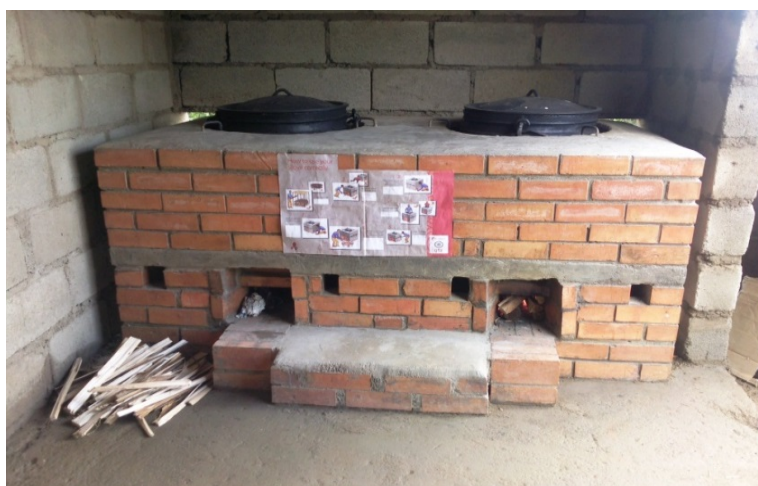
Figure 3.9: Libhubesi Cookstove at Orphanage Pre-School at Mahwalala
